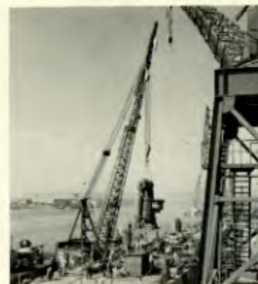
Boiler Emplacement, Sept. 1963
